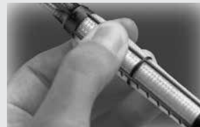
Step 2: Pierce the tip of the screen tube with the rod intended to be used to check embedment depth.
